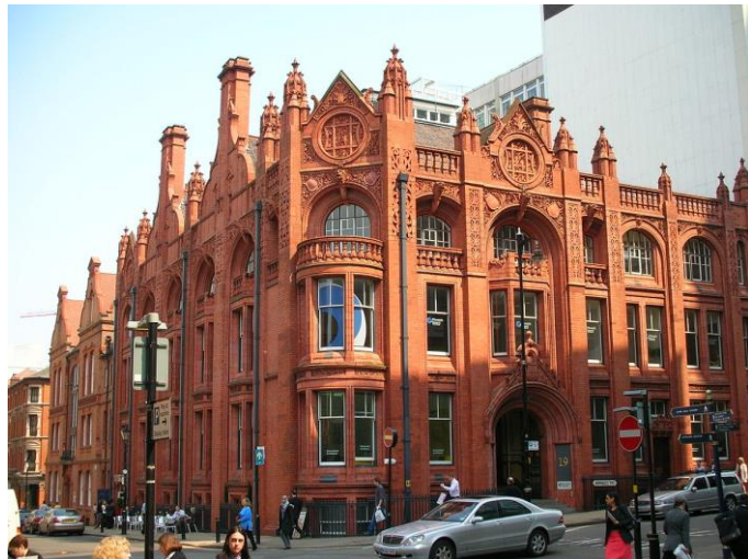
The Exchange Architectural terracotta Grade I listed building
